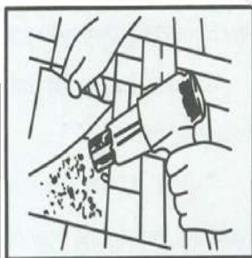
used for replacing the plastic tile
