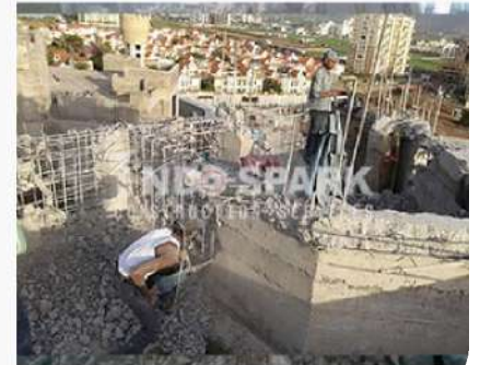
Breaking of Water Tank at Undri, Pune
