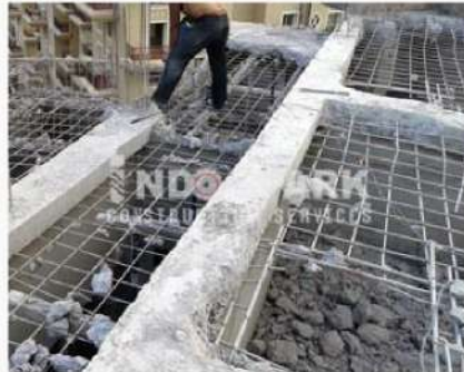
Breaking of Water Tank at Undri, Pune
