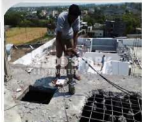
Concrete Splitting
