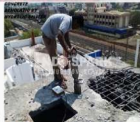
Concrete Demolition by Hydraulic Splitter
