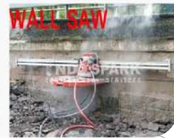
RCC Slab Cutting Work
