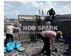
Removing cutouts by the help chainpullly
