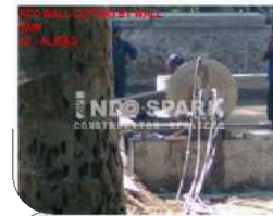
Removing cutouts by the help chainpullly
