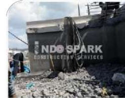
Removing cutouts by the help chainpullly
